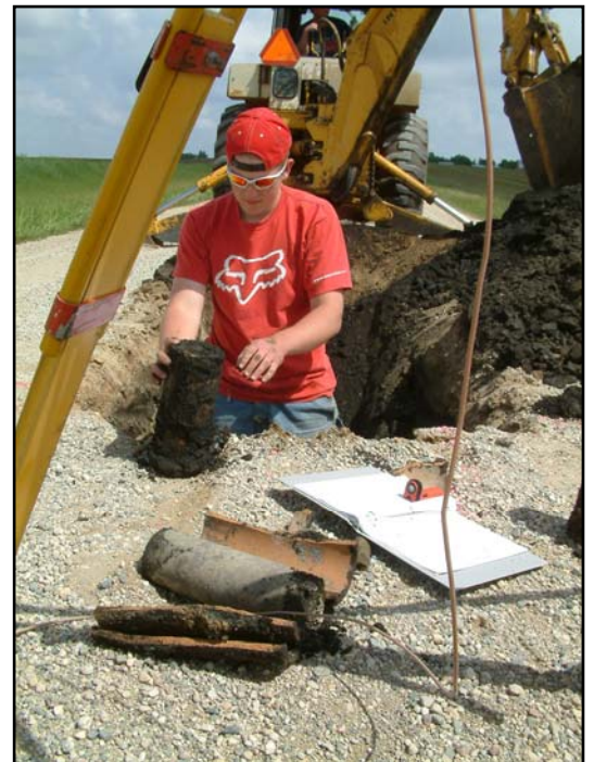
Bonnema Surveys Section Corner Recovery Efforts (the found section corner monuments lie in the foreground)
